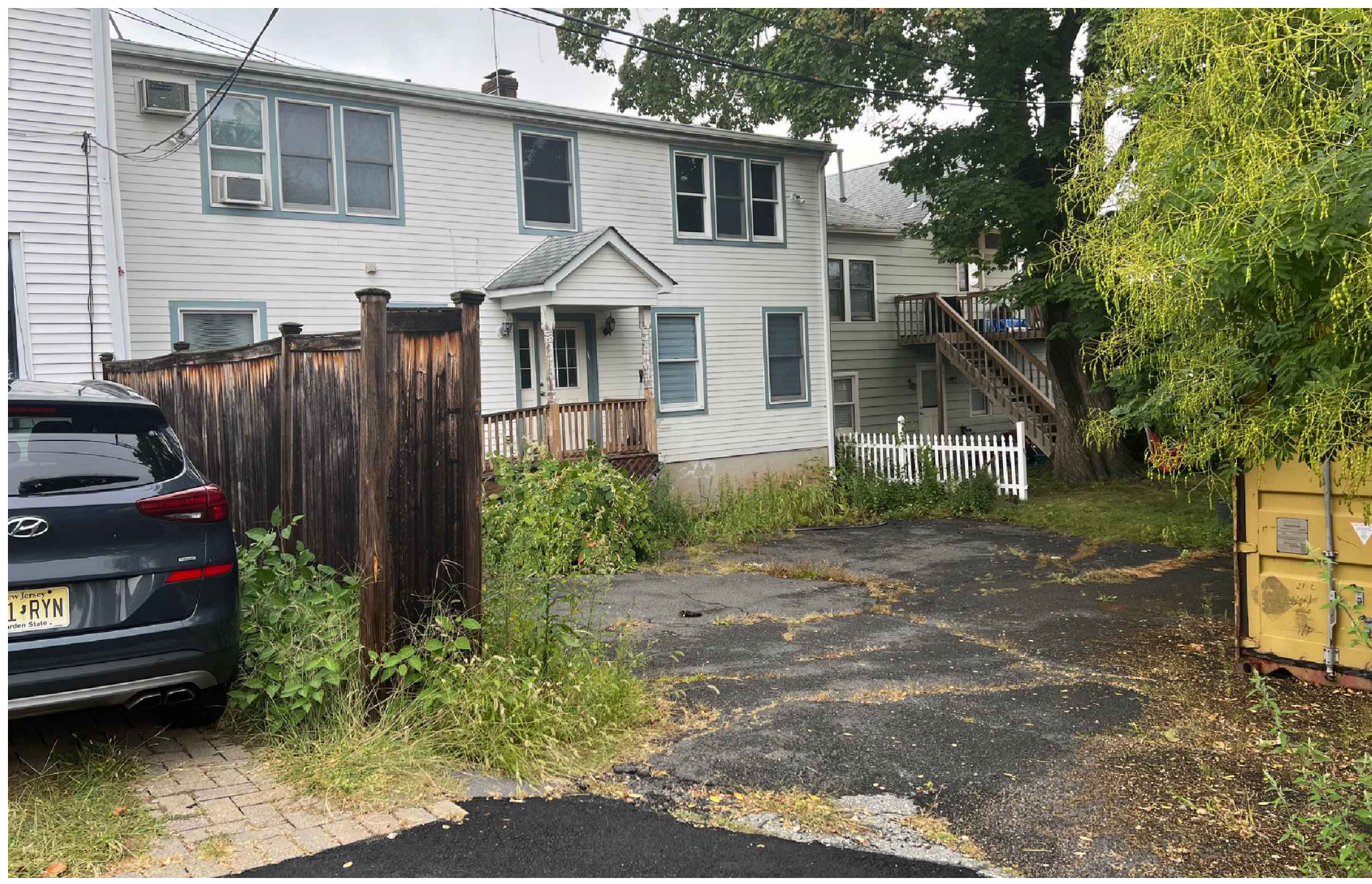
BURD STREET REAR FRONT VIEW LOT 3; BLOCK 3
