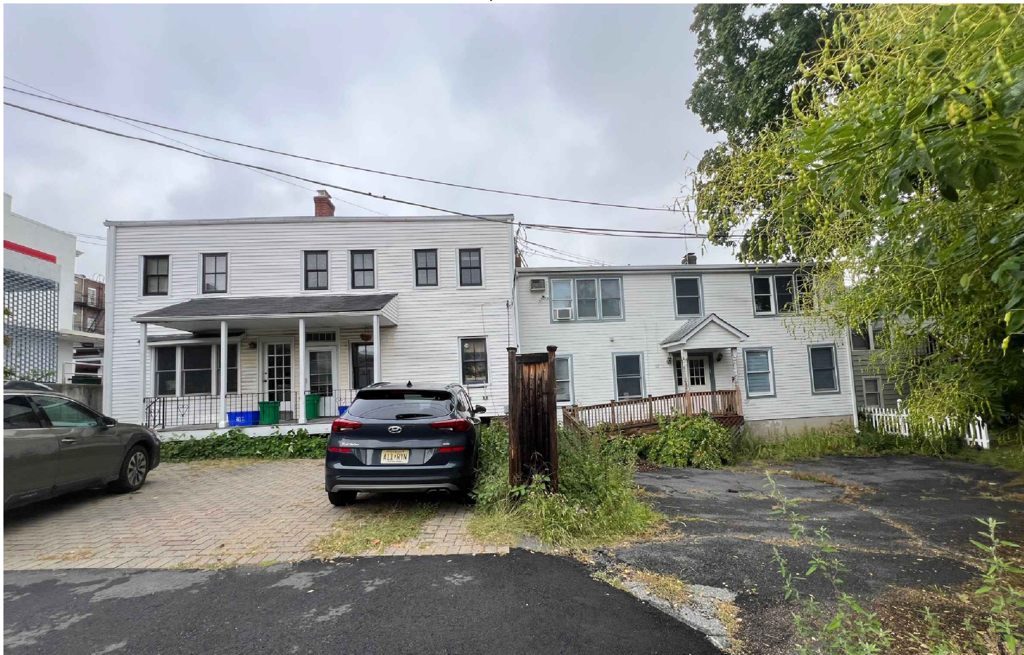
BURD STREET REAR LEFT VIEW LOT 2; BLOCK 3
